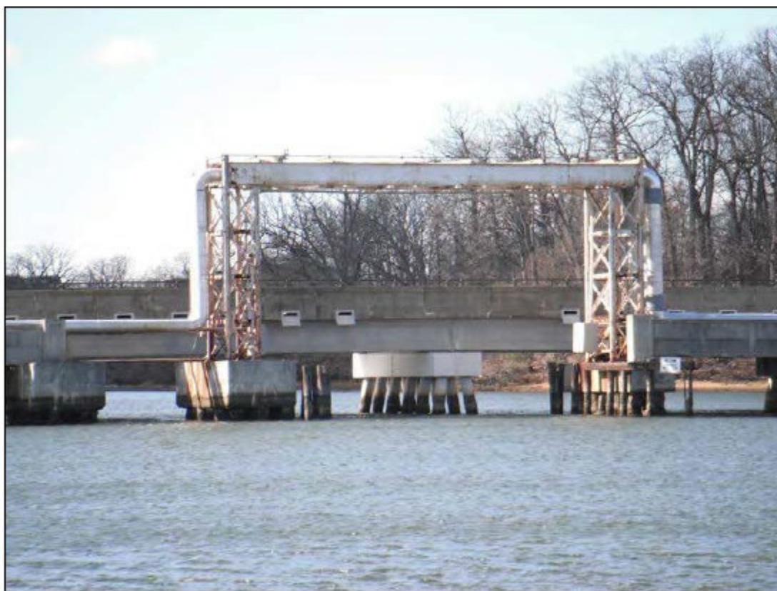
Figure 1-2: Utility Bridge, West View
